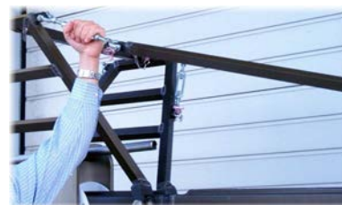
Tensioning the turnbuckle
